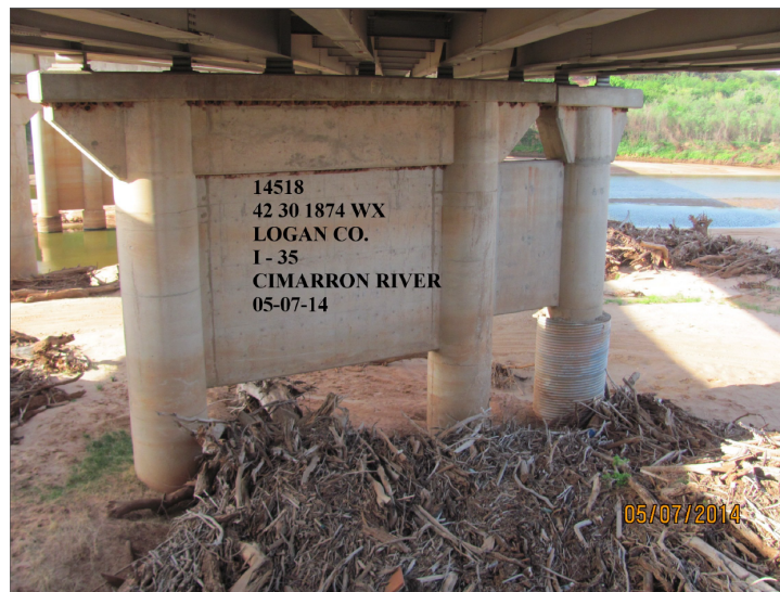
Figure 4.4: Photo of bridge substructure.
