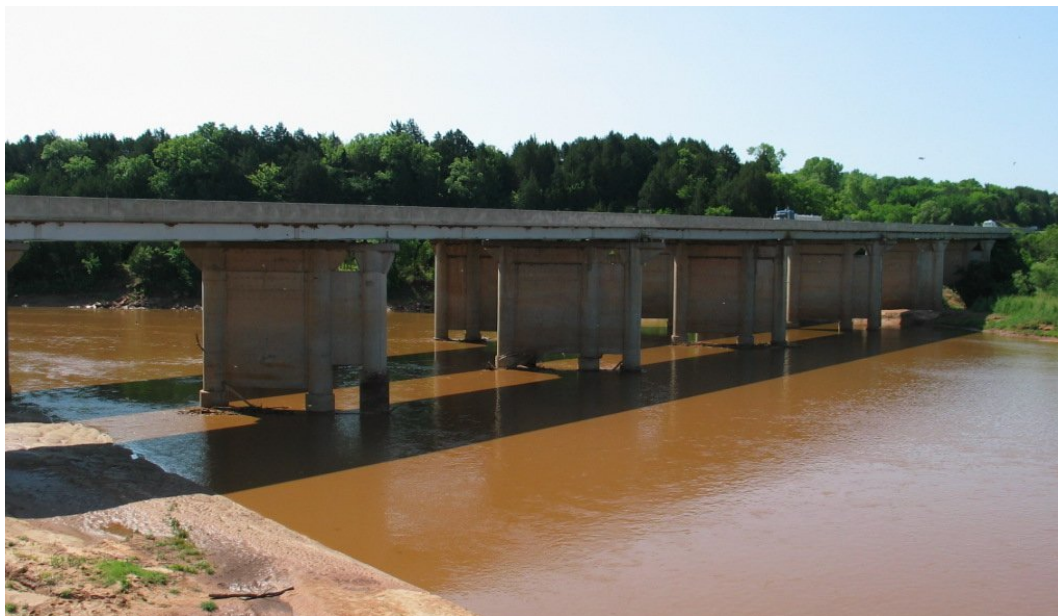
Figure 4.1: Photo of the I-35 bridge over the Cimarron River.
