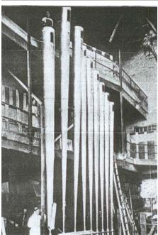
(Left) Recently uncovered archival picture from the Boston Herald on April 26, 1931, of the 32' Bombarde (M. P. Möller's first set of metal 32' pipes). The pipe on the left has a miter at the bottom so the pipe can fit under the 25' ceiling in the Philadelphia Municipal Auditorium. (Thank you to Barbara Owen for providing a copy of the clipping.)
