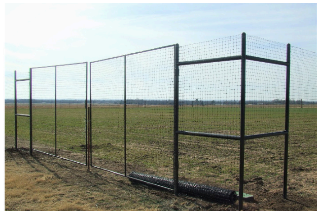
Wildlife exclusion fence. It is 8 feet tall.
