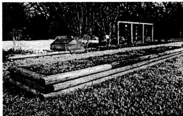
B. Reinforcing Rods Hold Timbers Together. Figure 3. Simple Landscaped Timber Raised Bed.
