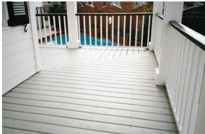
Figure 3. Application of wood plastic composites as decking.
