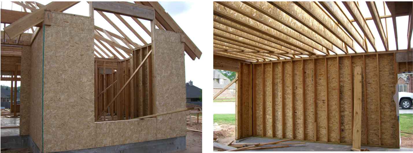
Figure 3. Applications of OSB as siding and I-joist
