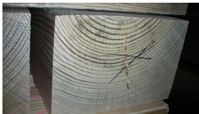
Figure 3. A deep crack on the cross-section.
