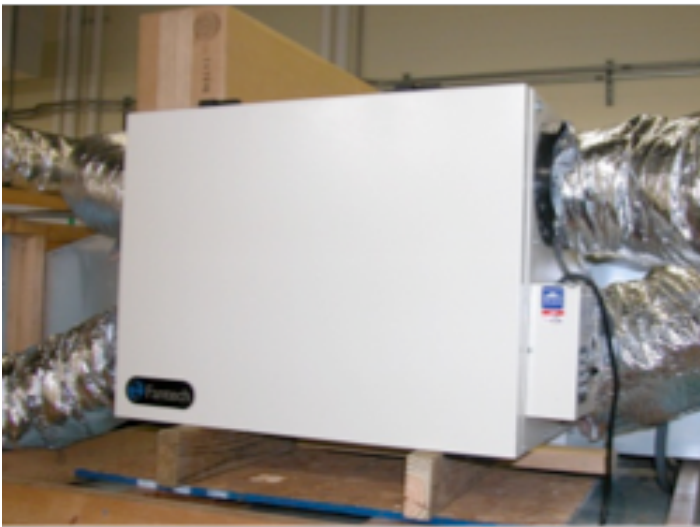
Figure 2. Typical VHR unit used to recover waste heat.
