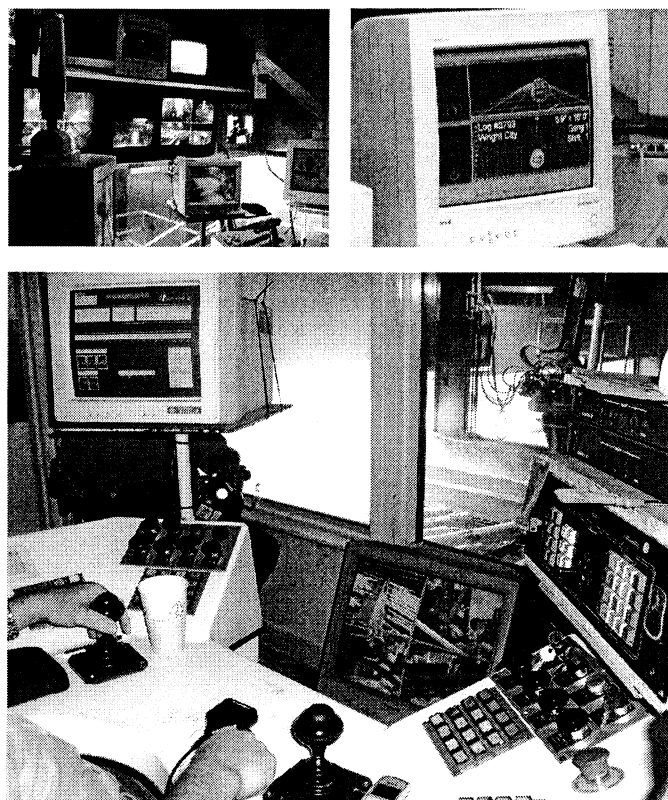
Figure 4. Primary breakdown of logs: headrig control room. (Courtesy of Weyerhaeuser Inc.)
