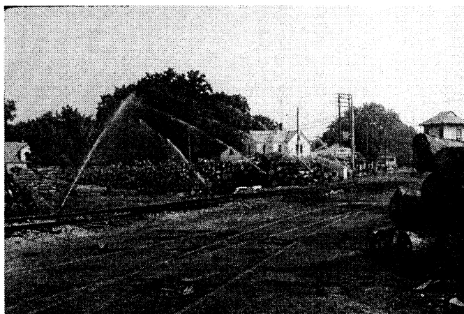
Figure 1. Sprinkler system to keep logs in wet condition.
