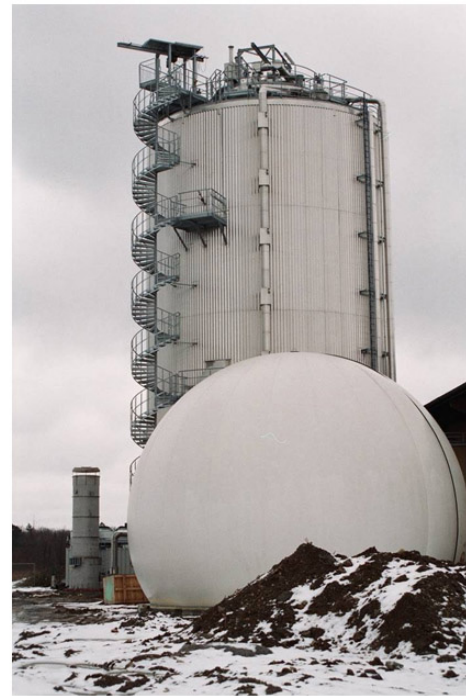
Figure 5. A DRANCO single phase silo reactor used to digest solid municipal waste in Germany (from www.tkm.sebe.eu ). Sphere in foreground is biogas storage.
