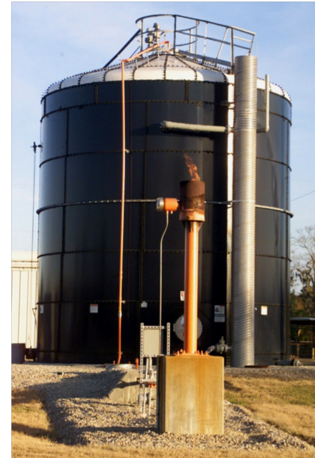
Figure 8. Fixed film digester located on the University of Florida Dairy Research Farm (Photo courtesy of Ann Wilkie, University of Florida).
