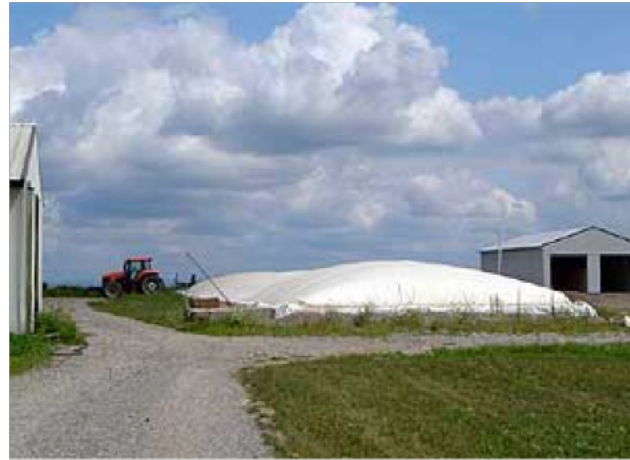
Figure 5. Plug flow digester located on the Emerling Farm in Perry, N.Y. (Photo courtesy of Cornell University/USEPA).
