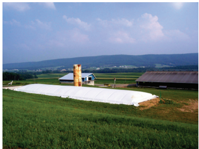
Figure 5. Plug Flow Digester on a Dairy Farm (from www.RCMdigesters.com ).
