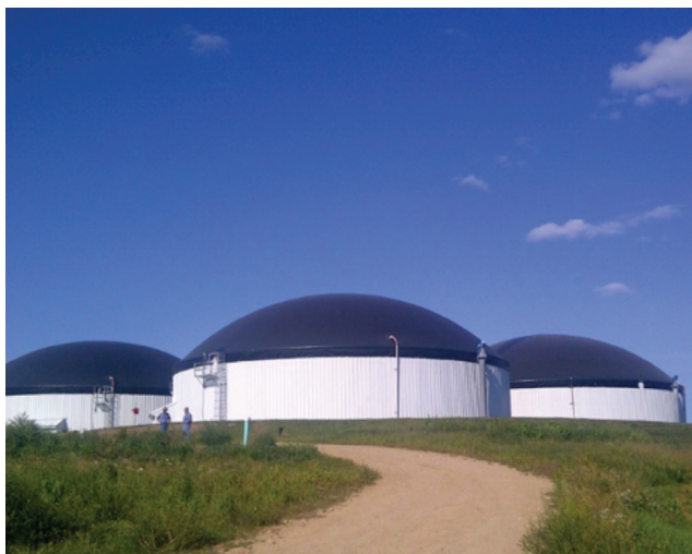
Figure 3. Three Complete Mix Reactors making up the Dane County Community Digester near Madison, Wisconsin.
