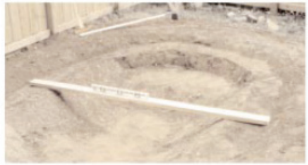
Leveling the pond during construction.
