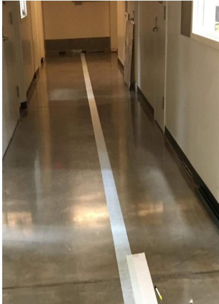
Figure 4-8 - Web Spread on the Floor
