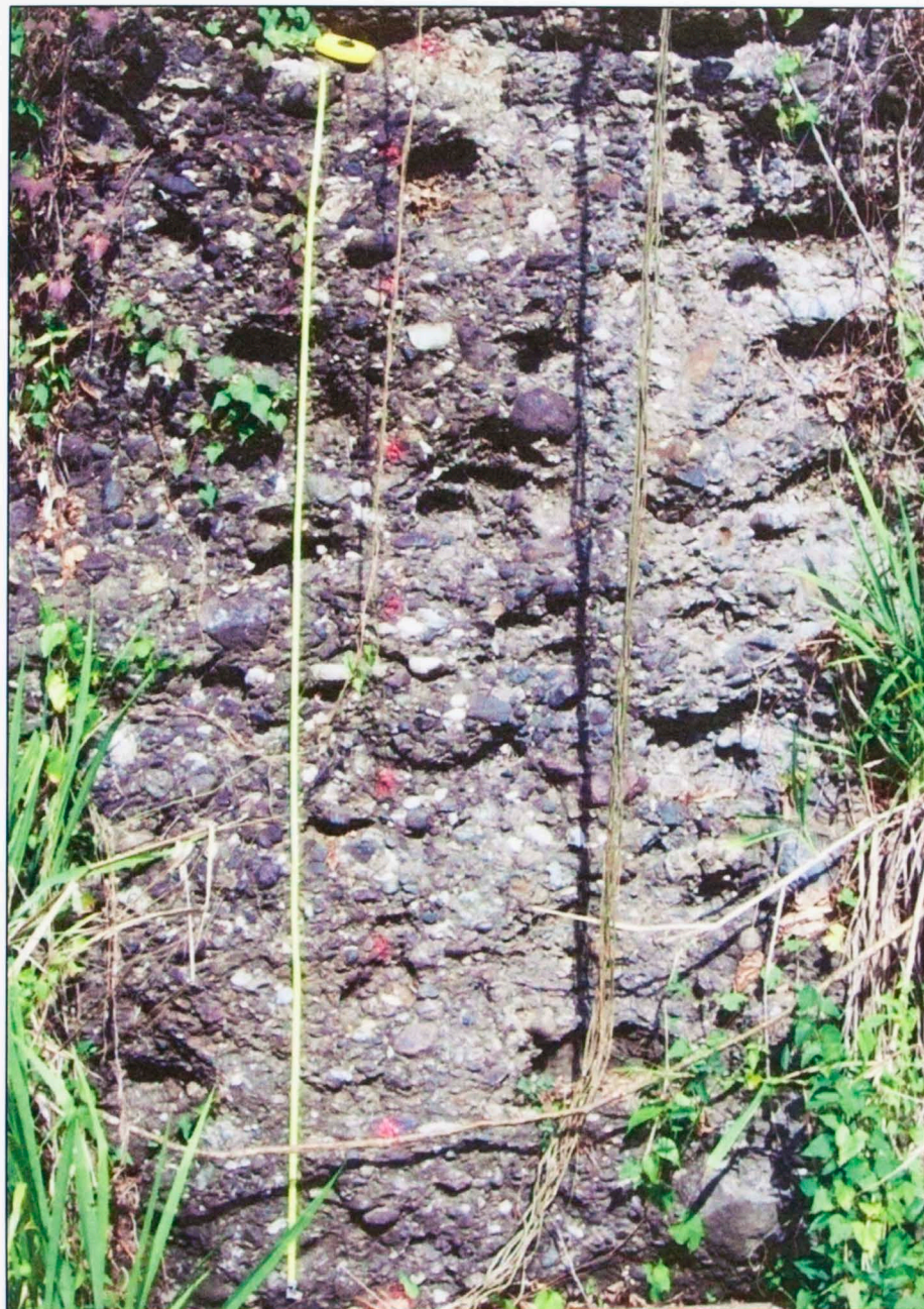
Figure 2.4.3: Albany Member of the Richmond Formation along highway A3 between Whitehall and Albany. It is composed of massive, very poorly sorted conglomerates with a sandy mudstone matrix. The beds are clast-supported, but appear matrix-supported. The painted red dots can be used for scale. Each represents one foot in measurement (Wescott and Ethridge, 1983).
