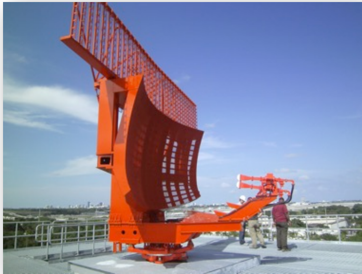
Figure 2.3: S-band ASR antenna (courtesy of Wiley/Wilson). This antenna produces a beam that is narrow in the azimuth dimension and wide in elevation dimension, which is commonly referred to as a “fan” beam. By having a wide beamwidth in elevation, the radar can complete a volume scan by only rotate in azimuth. This allows for faster updates but the position of the target in elevation cannot be accurately estimated.
