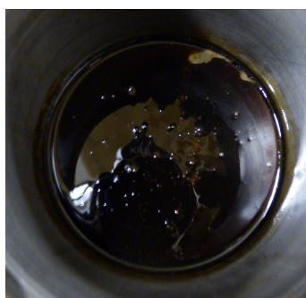
Fluid in accumulator
