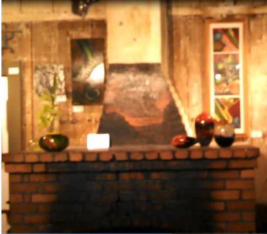
Figure 3.11 – Fireplace and Chimney, Volcano House
