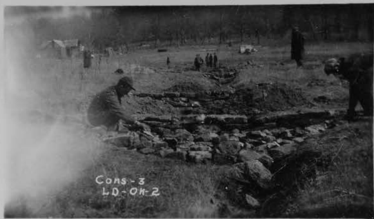
Picture No. 39 Check dams built of native stone.
