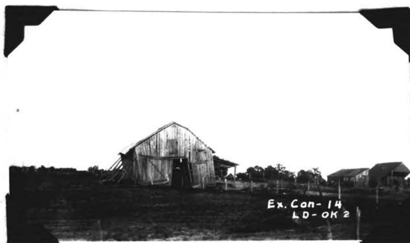
Farm buildings in a run-down condition
