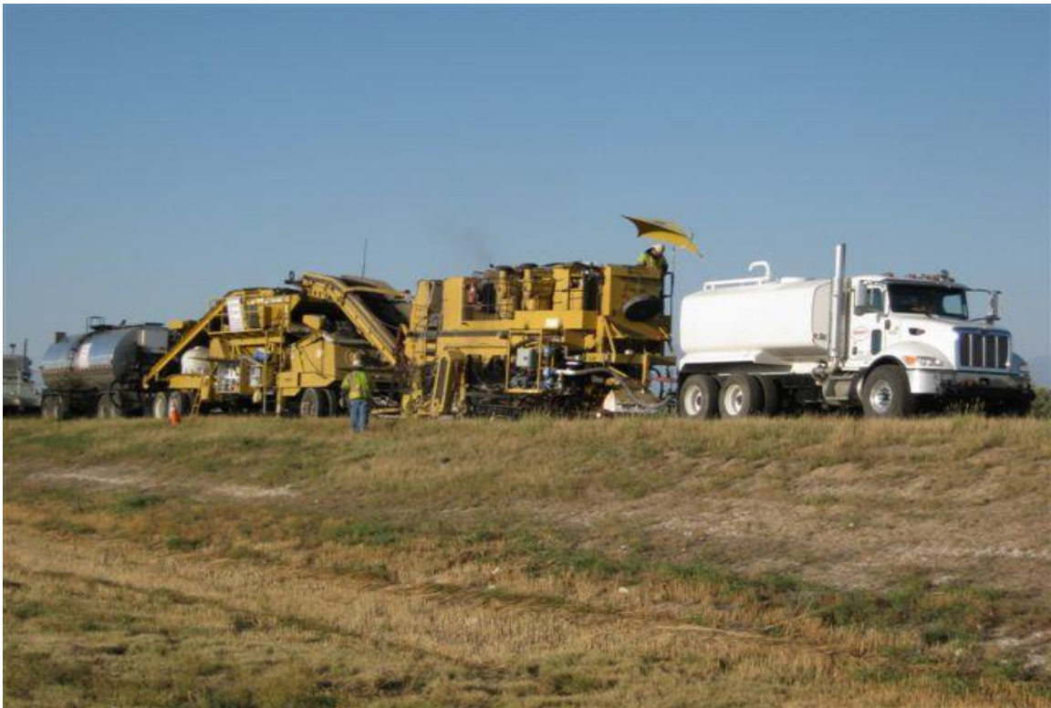
FIGURE 4 Cold In-Place Recycling equipment
