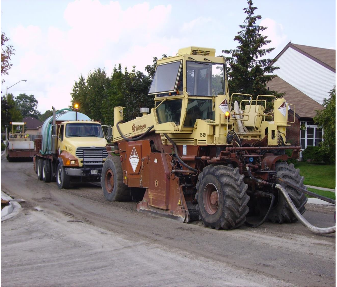
FIGURE 2 Full depth reclamation unit
