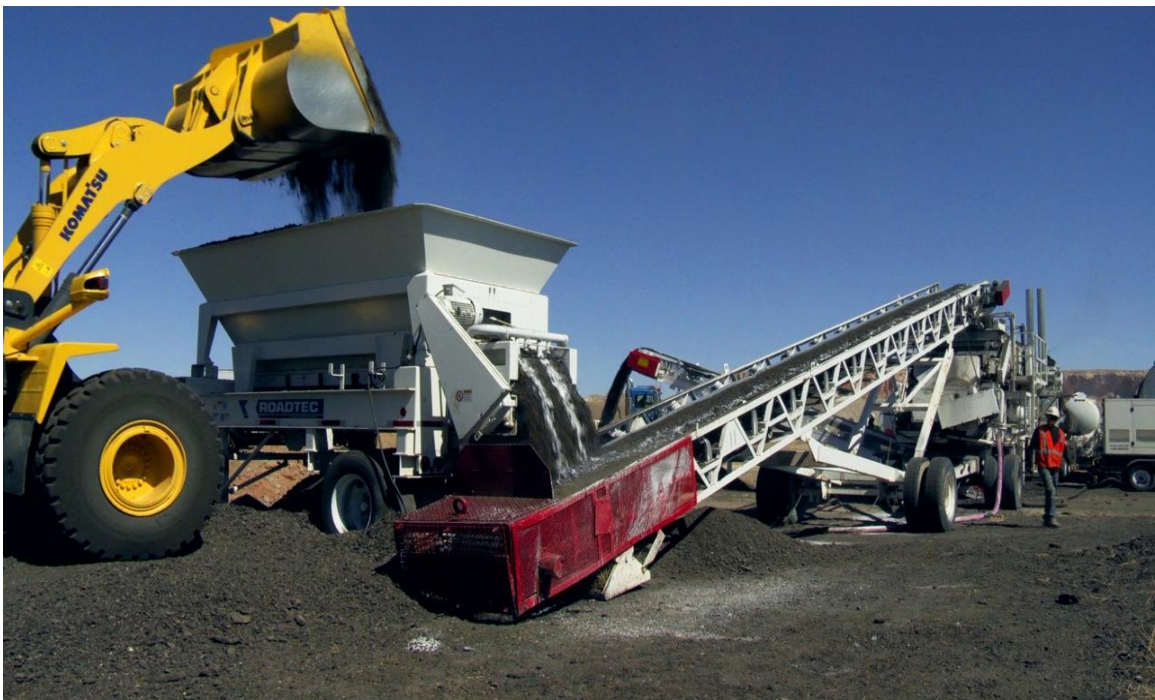
FIGURE 3 Cold central plant recycling
