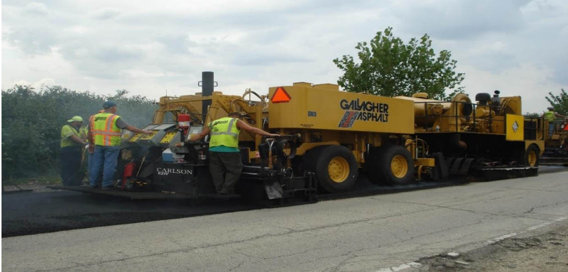
FIGURE 1 Hot in-place recycling unit
