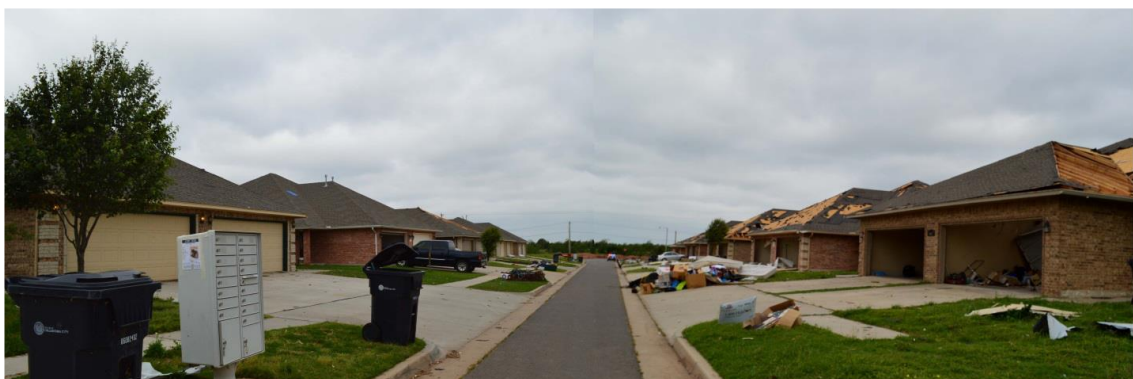
Figure 1-6 Failure of Garage Doors (Tornado Damage Assessment in the aftermath of the May 20th 2013 Moore Oklahoma Tornado, 2014)
