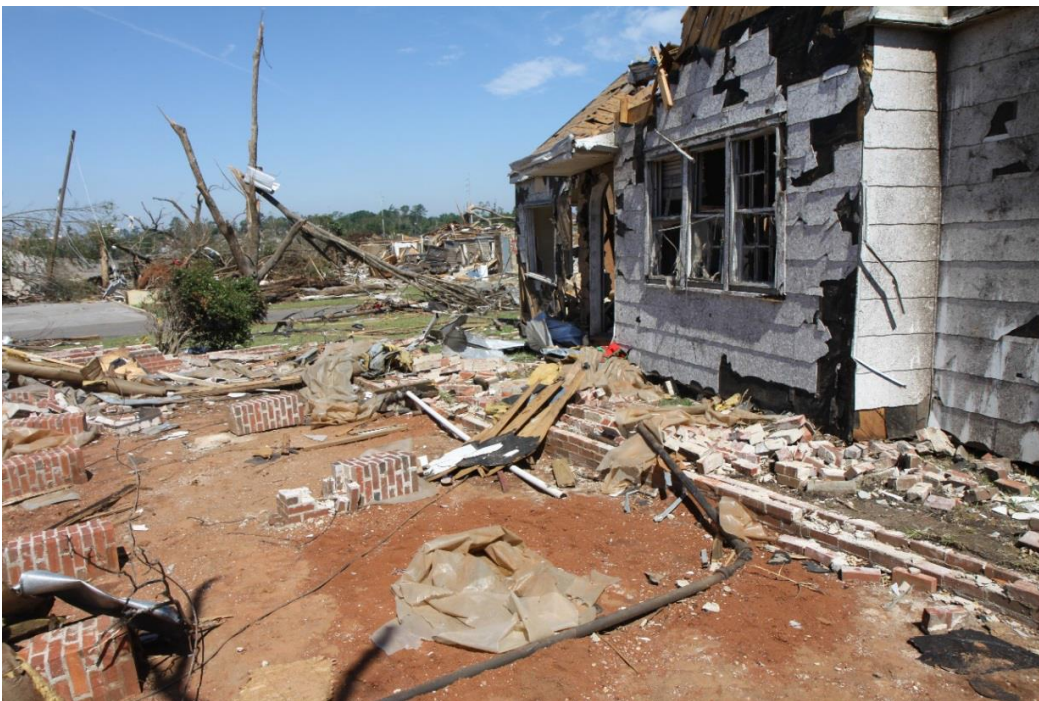
Figure 1-19 House shifted off of crawlspace foundation in Tuscaloosa, AL after 2011 Tornado. (Tornado Damage Assessment in the aftermath of the May 20th 2013 Moore Oklahoma Tornado, 2014)
