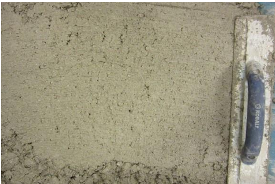
Fig. 1-5 shows a float finishing the surface of the concrete.
