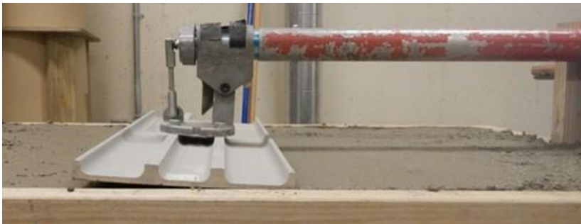
Fig. 6-2 shows the bull-float being used.
