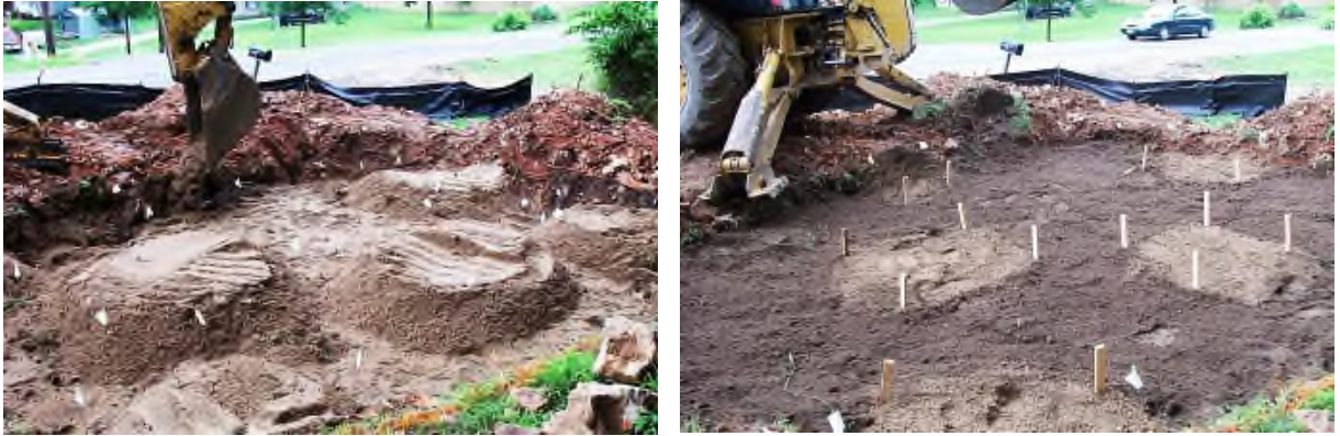
Figure 2- 5. Sand plug construction.
