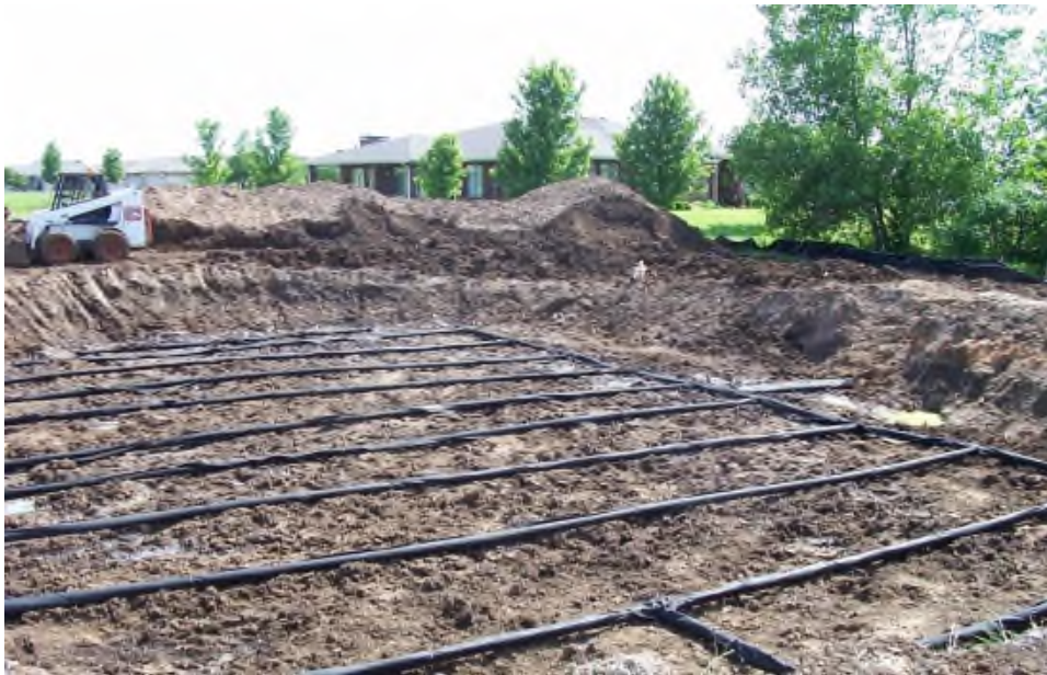
Figure 2- 4. Cell drainage pipe layout.
