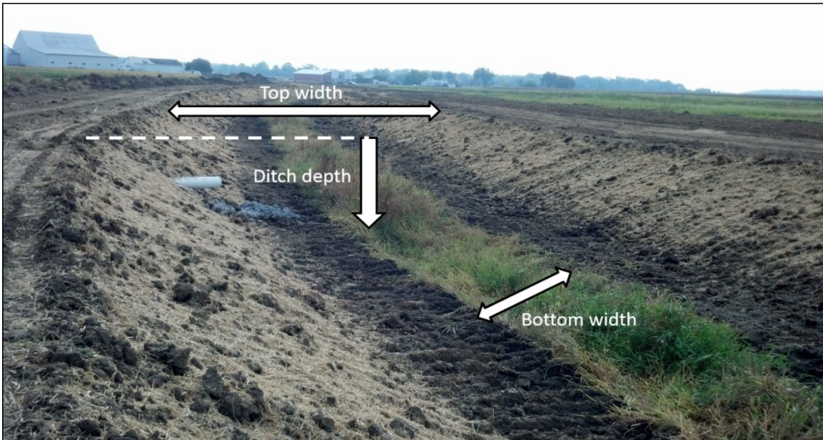
Figure 4.7. A drainage ditch fed by a tile drained agricultural field in Ohio is shown with top width, bottom width, and depth marked.
