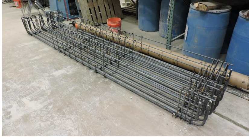
Figure 4.3: Completed Reinforcing Cage
