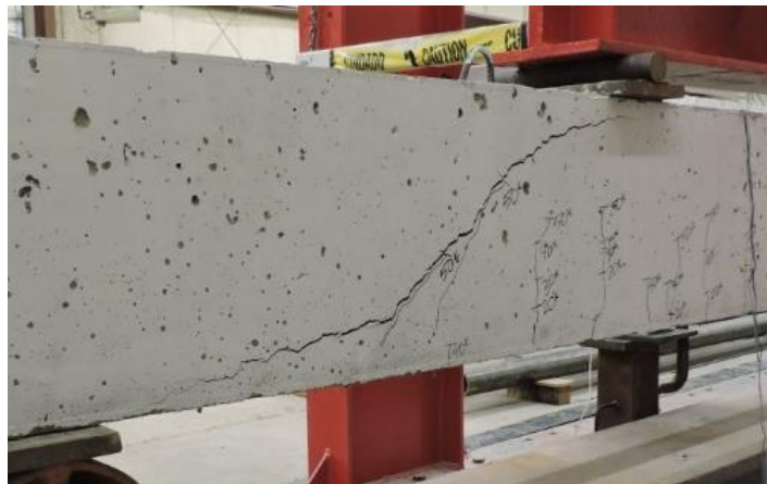
(c) K-E1-3 Failure Crack
