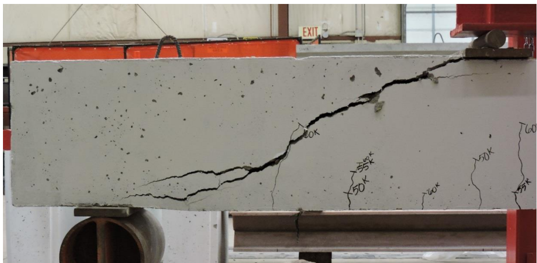
Figure 4.14: Shear Failure Example
