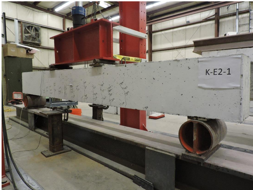
Figure C.4: K-E2-1 Crack Propagation 50 kips
