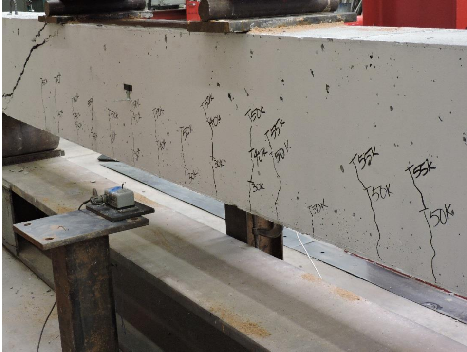
Figure A.17: K-C-3 Failure Crack Right View
