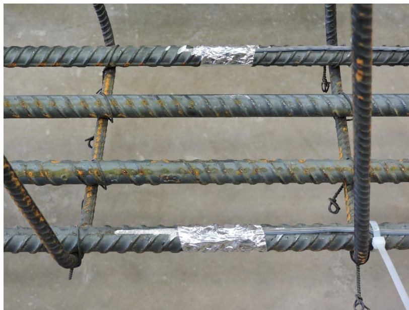
Figure 4.6: Completed Strain Gauges
