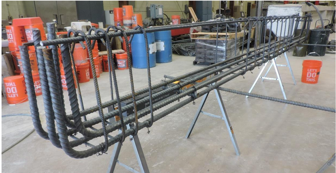
Figure 4.4: Completed Reinforcing Cage
