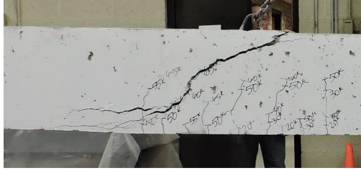
(a) K-E1-1 Failure Crack
