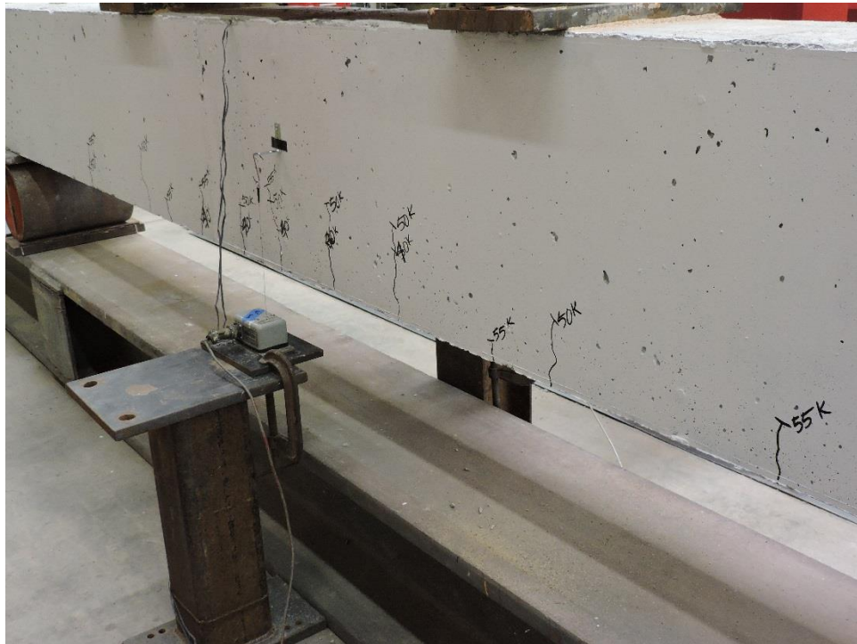
Figure A.2: K-C-1 Crack Propagation 55 kips
