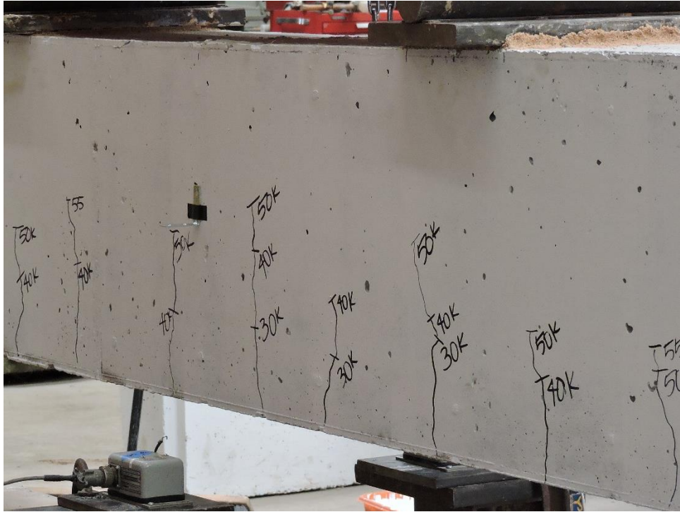
Figure A.9: K-C-2 Crack Propagation 50 kips
