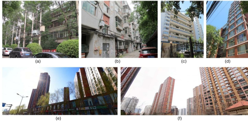
Figure 46 Building Conditions in Liu Pu Kang and Sun Palace Communities
