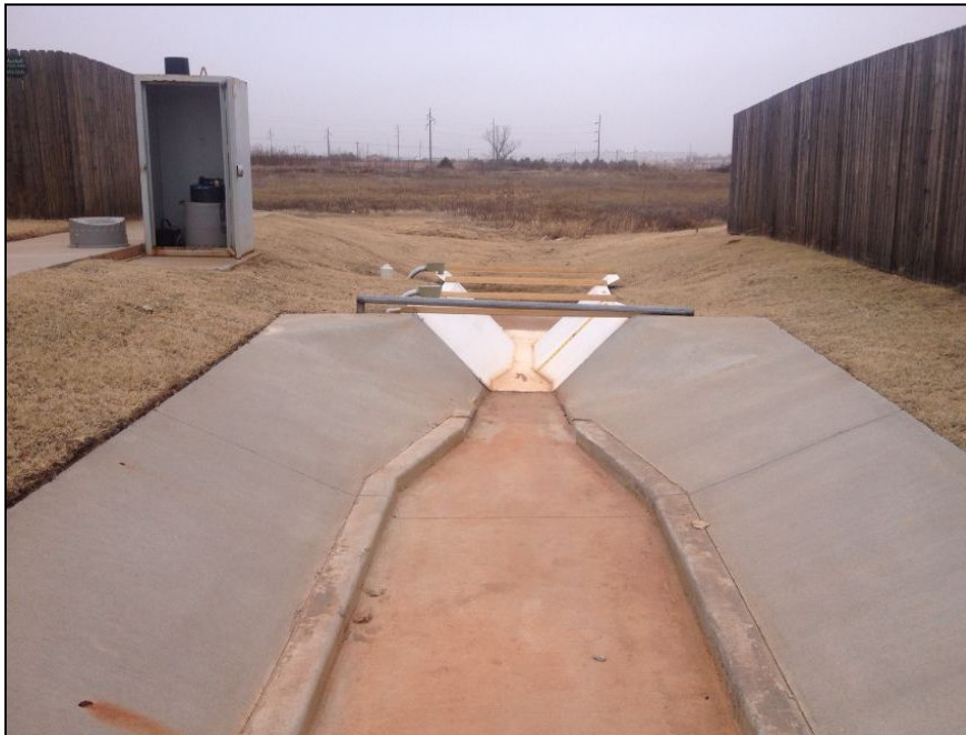
Figure 5. Flume and autosampler installation at Trailwoods (TW) treatment watershed
