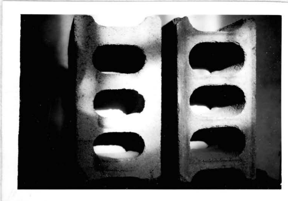
Fig. 7 - Opposite Core Ends of Sand and Gravel Aggregate Concrete Block Used in Walls of Temperature-Controlled Shelter.
