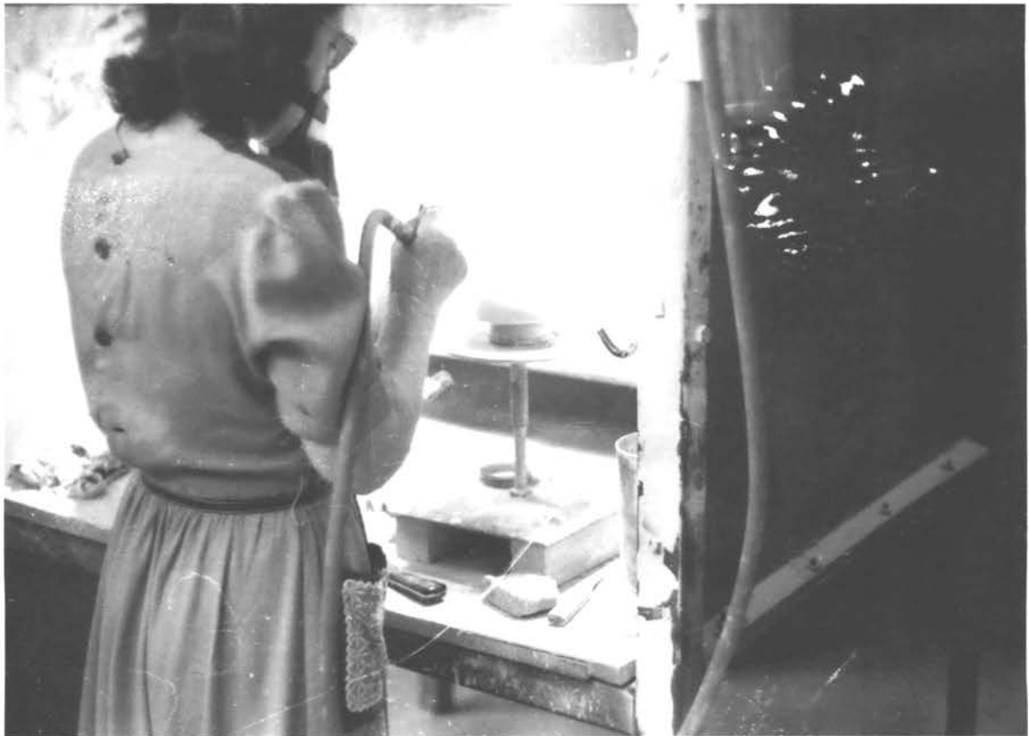
Applying trimming coat of glaze.
