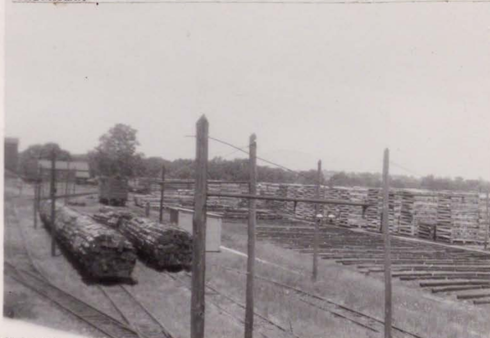
Fig. 18b. Frisco Storage Yard adjoining the Creosoting Plant. Ties are stored in this yard to await the creosoting process. The yard is interlain with narrow tracks.
