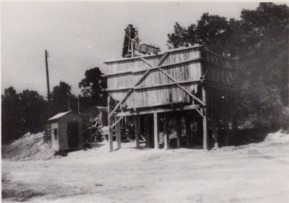
Fig. 19a. Crusher and Hopper at the Choctaw Lime Company lime plant near Fort Towson, Oklahoma. Lime rock is dumped into the crusher (to the left of the hopper) and crushed, then the conveyor chain hoists the crushed lime into the hopper. Trucks back under the two hoppers to be loaded.
