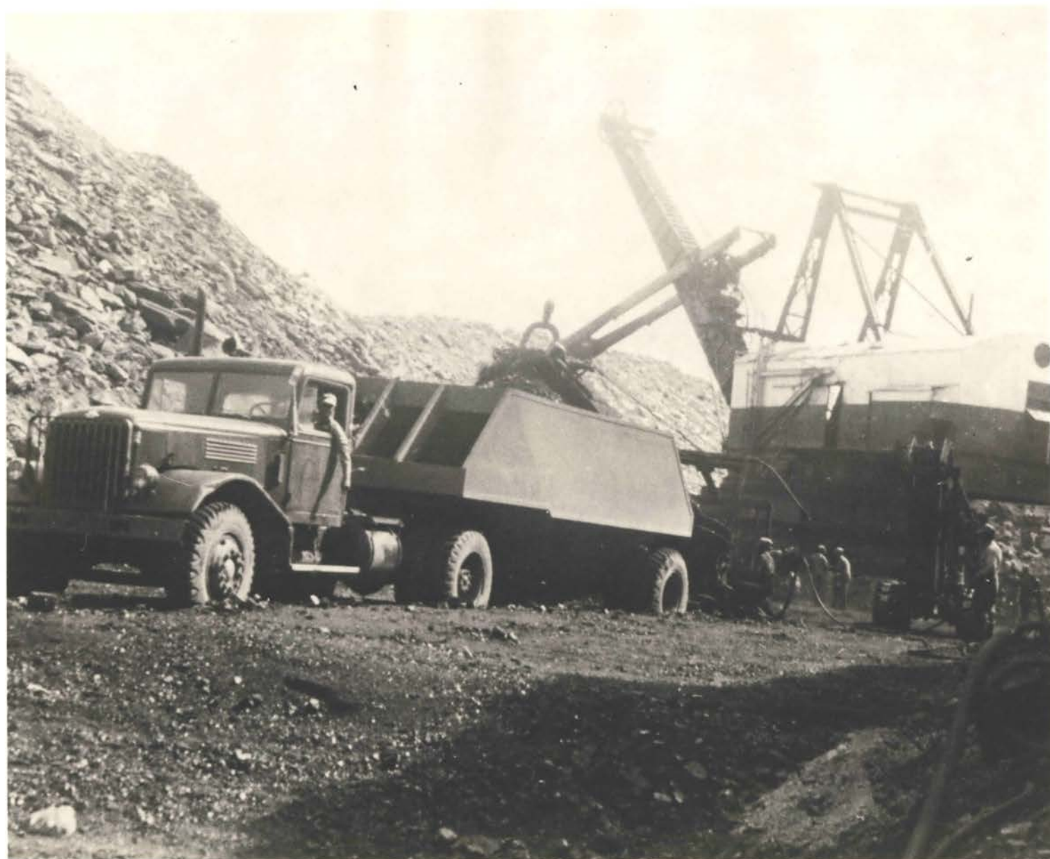
STRIPPING OPERATIONS FIGURE 4
