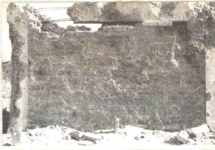
FIGURE 31. TWELVE INCH BRICK WALL AFTER SUBJECTED TO BOMB BLAST be designed with any degree of certainty.
