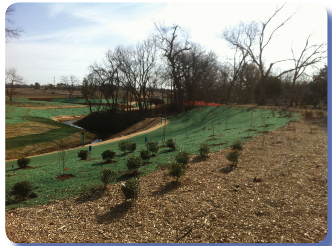
Picture above: Progress shown at Cow Creek.
