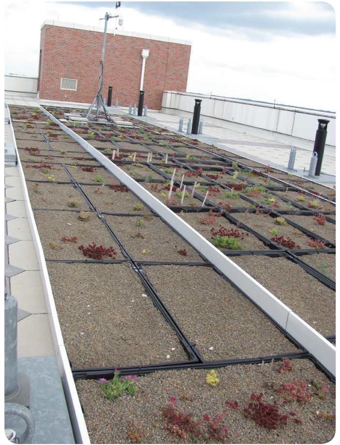
Figure 2: Experimental green roof at the National Weather Center in Norman.
