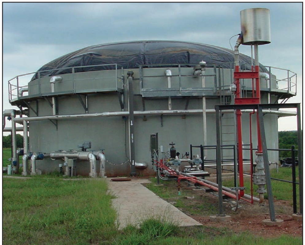
Anaerobic digester producing biogas from swine manure at the OSU Swine Research and Education Center.
