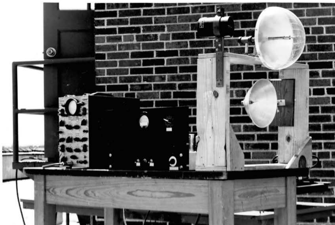
Figure 5 (A) Transmitting and Receiving Antennas
