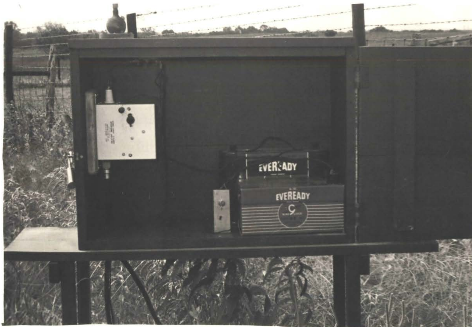
Figure 5. Antenna to coaxial line cathode follower with power supply.
