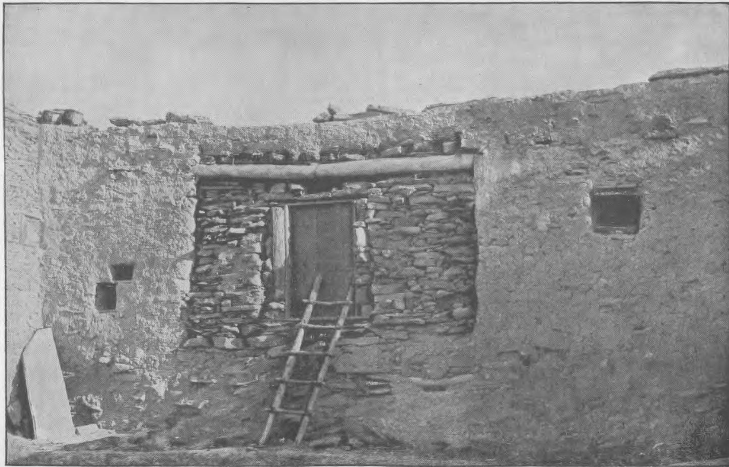
PARTIAL FILLING-IN OF A LARGE OPENING IN ORAIBI, CONVERTING IT INTO A DOORWAY.
