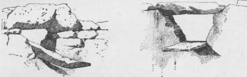
FIG. 39. Single stone roof drains.
