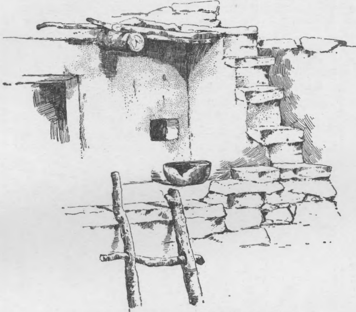
FIG. 48. Stone steps at Oraibi, with platform at corner.
