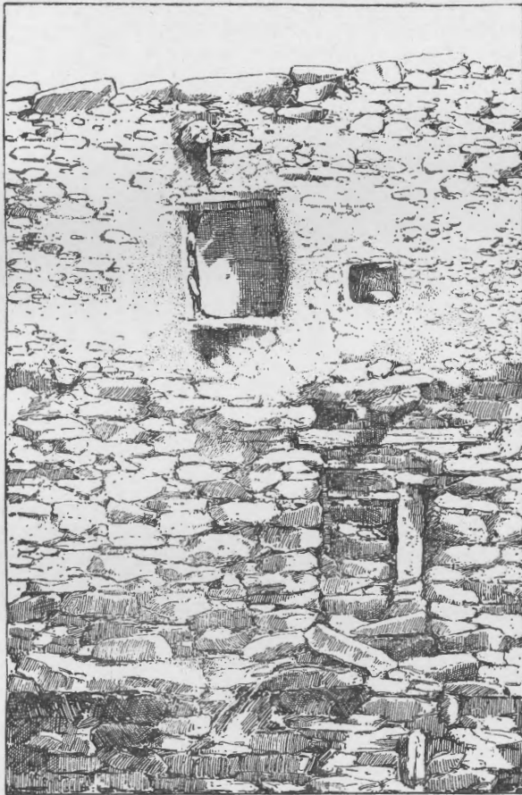
FIG. 92. Sealed openings in Tusayan.
