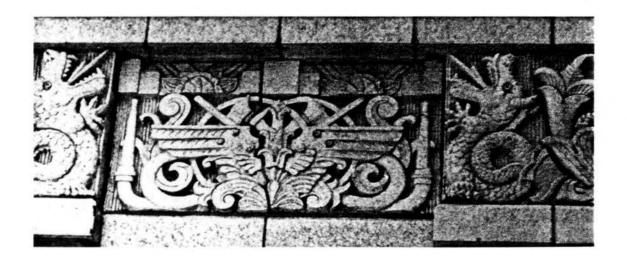
Figure 28. Terra cotta detailing above front windows
