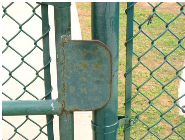
Image 3.37 Gate detail Denton, TX
