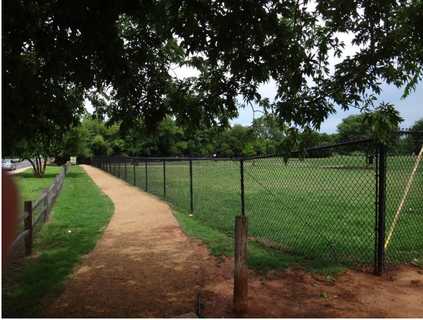
Image 3.23 Walkway entrance Edmond, OK
