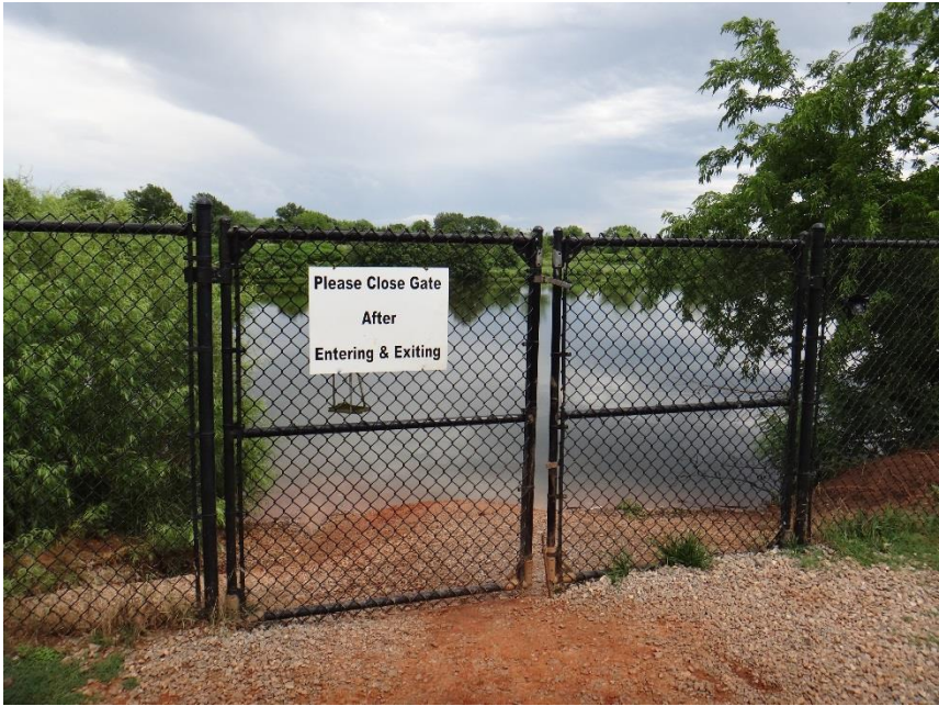
Image 3.22 Pond access Edmond, OK
