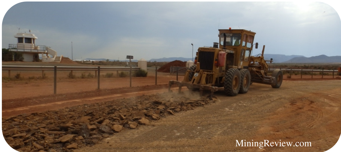
Figure 1: Example of Scarifying the Subgrade
