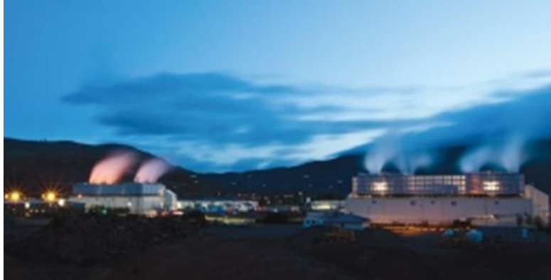
Figure 1 Steam carries heat away from Google’s data center in The Dalles, Oregon [5]
