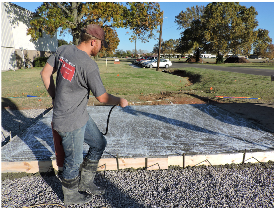
Figure 7.26 - Applying Sealant to the Finished Pavement
