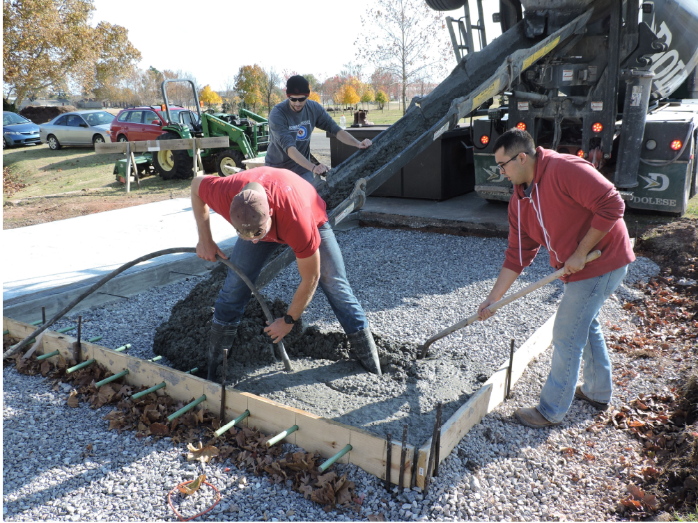
Figure 7.19 - Vibrating to Consolidate the Fresh Concrete
