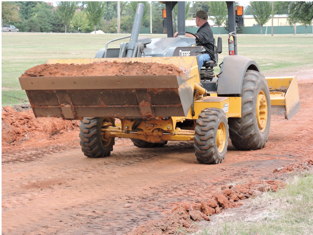
Figure 7.12 - Excavation of the Existing Subgrade
