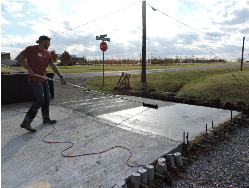
Figure 7.25 - Broom Finish on the Concrete Panel
