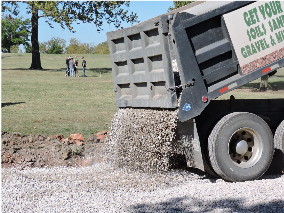
Figure 7.13 - Field Implementation Aggregate Base Placement
