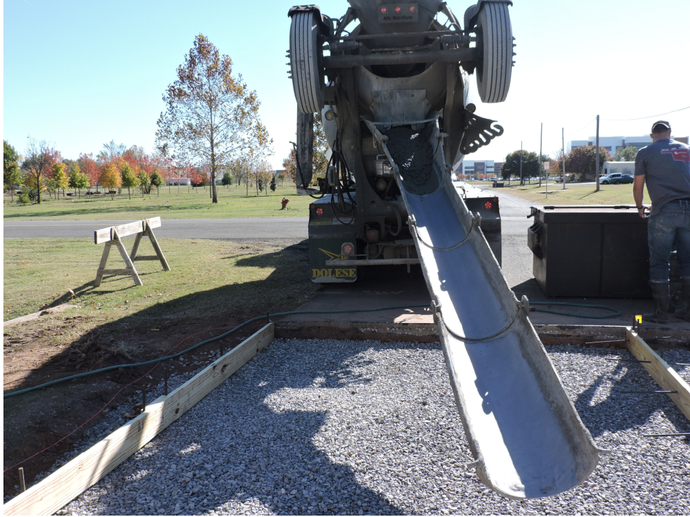
Figure 7.17 - Concrete Placement using Ready-Mix Truck
