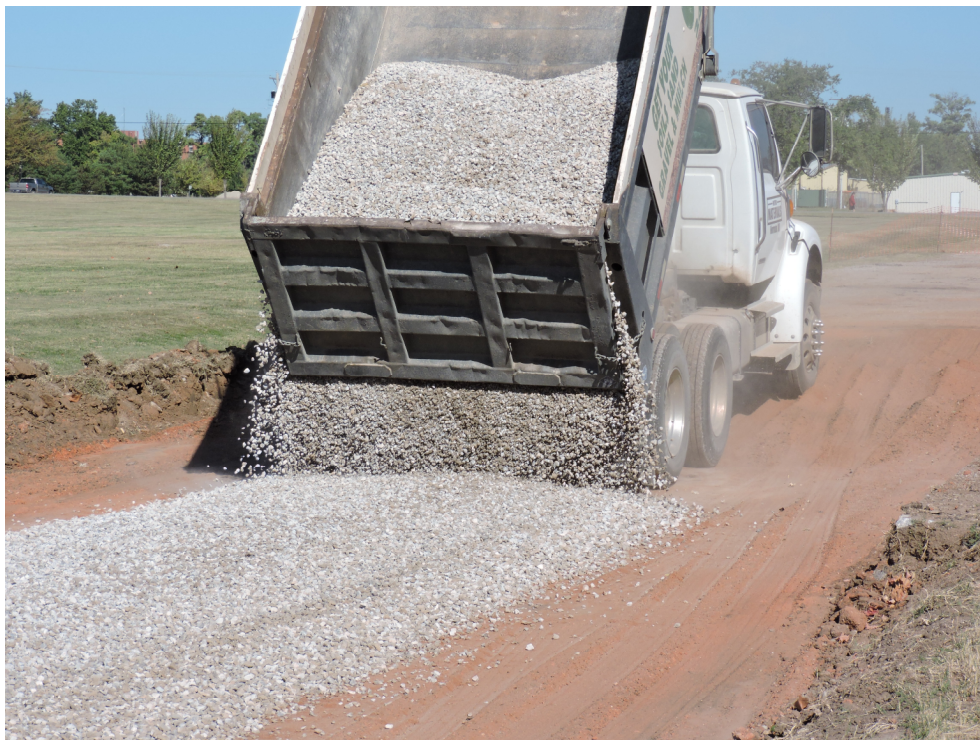
Figure 7.14 - Field Implementation Aggregate Base Placement
