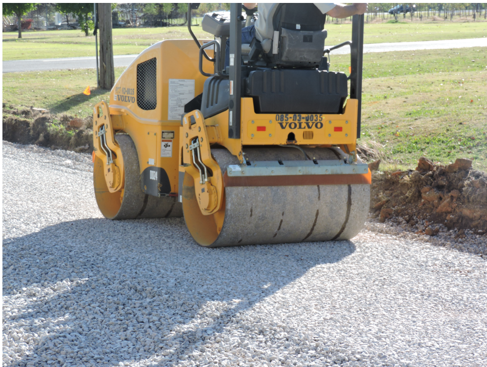
Figure 7.16 - Compaction of the Aggregate Base Using Vibratory Roller
