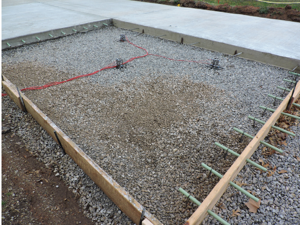
Figure 7.10 - VSWG Tree placement of in an Instrumented Panel
