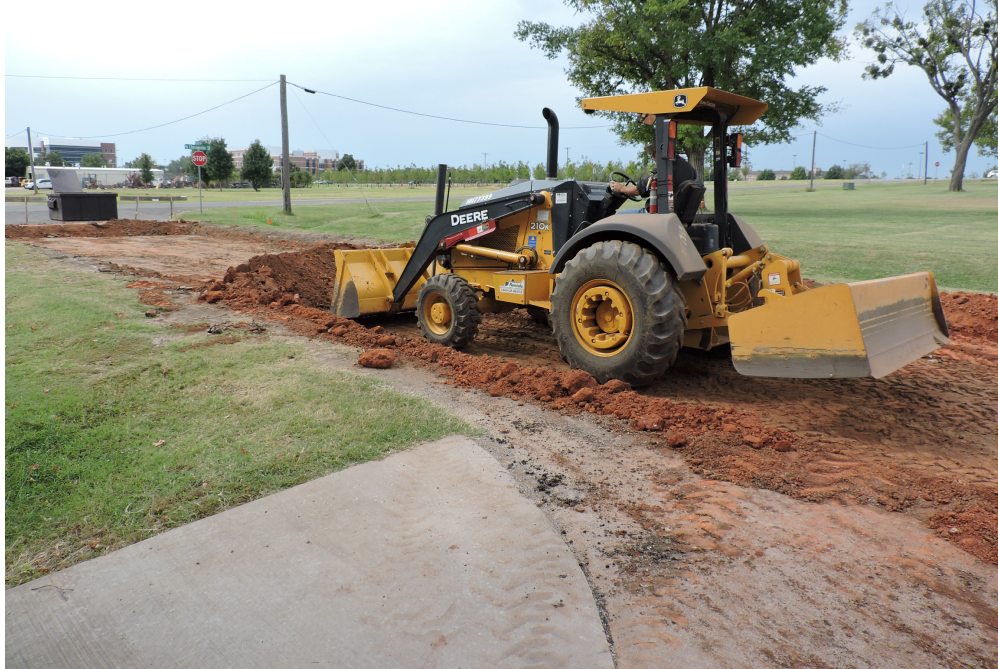
Figure 7.11 - Excavation of the Existing Asphalt and Subgrade
