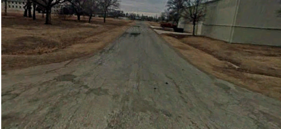
Figure 7.1 - Existing Asphalt Pavement
