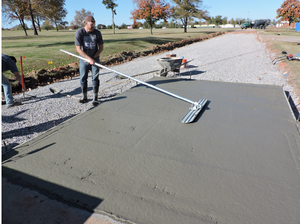
Figure 7.23 - Using the Bull Float
