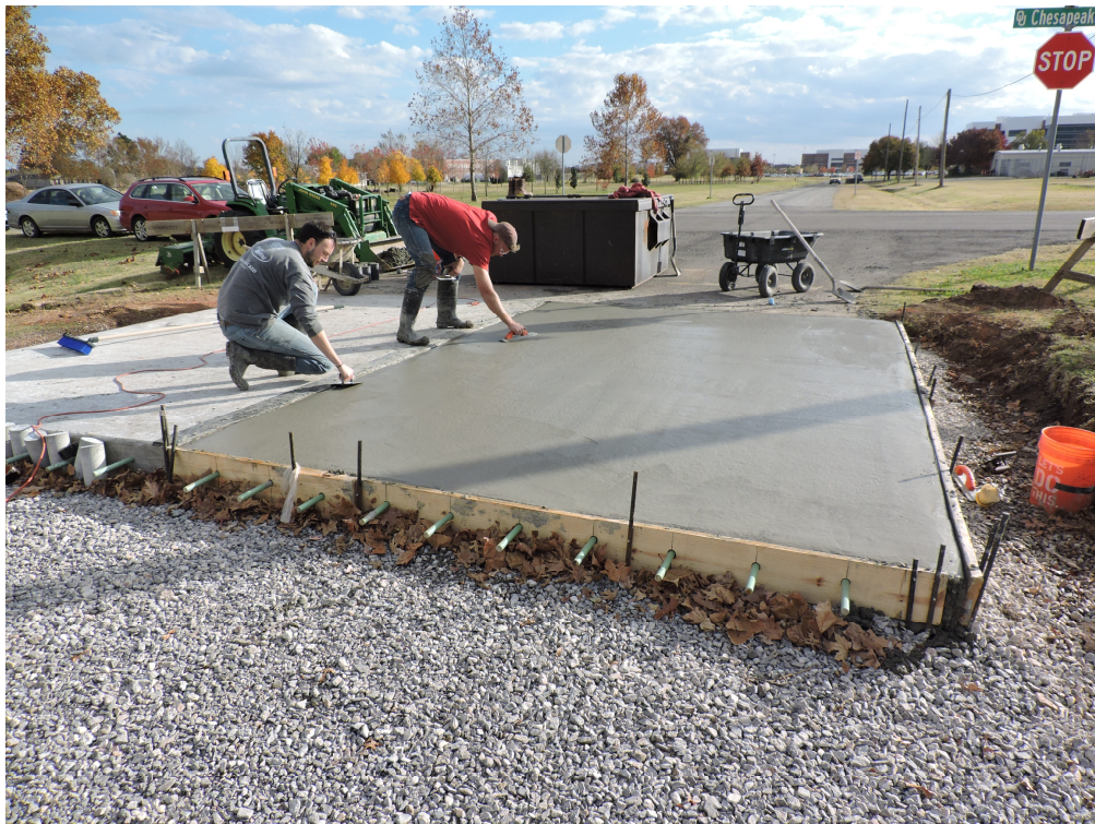
Figure 7.24 - Hand Floating and Edging the Panel
