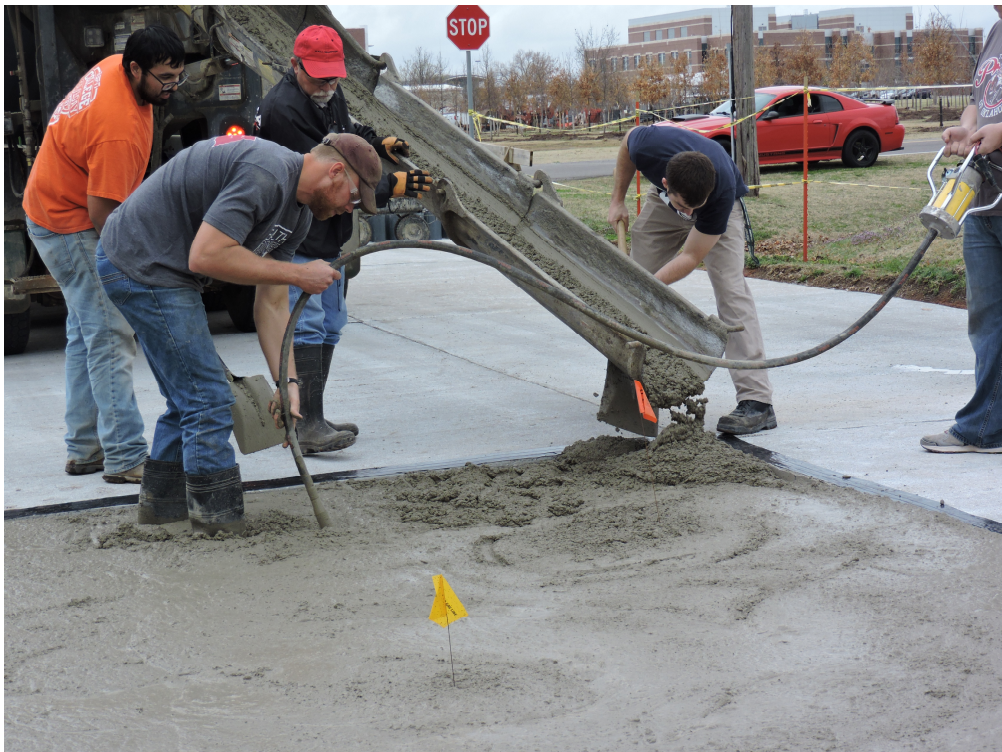
Figure 7.20 - Vibrating the Fresh Concrete
