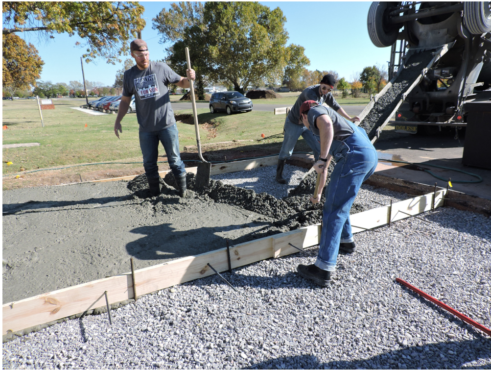
Figure 7.18 - Spreading and Leveling the Concrete with Shovels
