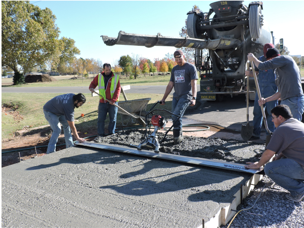
Figure 7.21 - Screeding for Final Leveling of the Concrete
