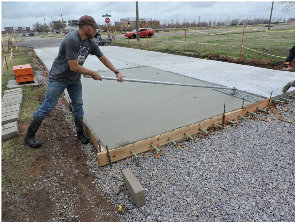
Figure 7.22 - Floating the Center of Panel
