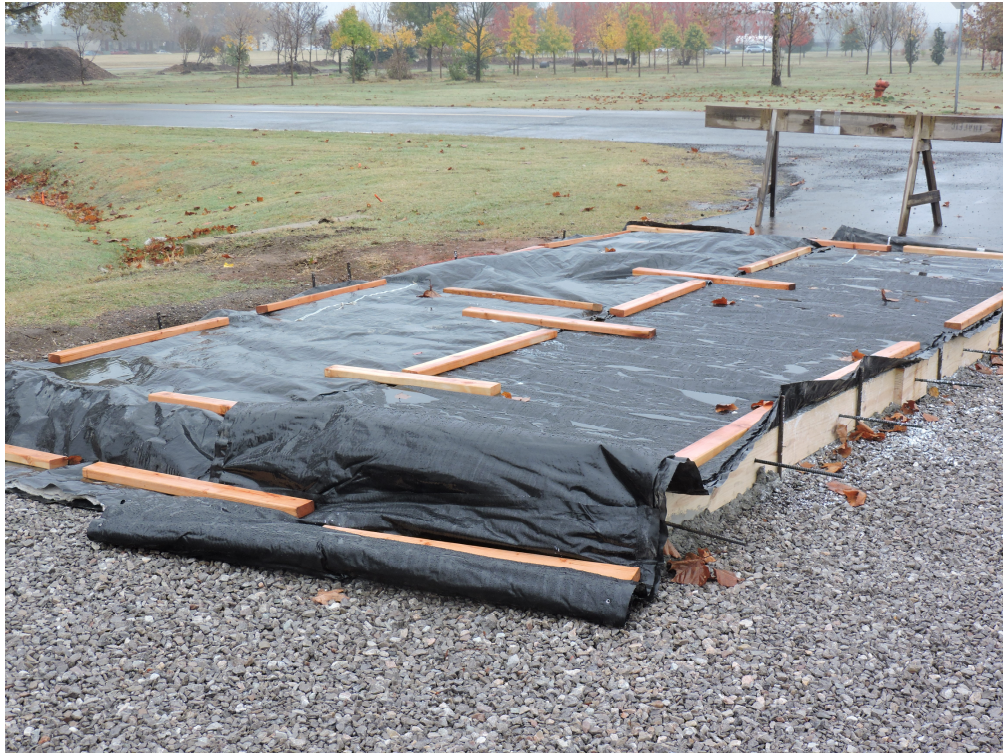
Figure 7.27 - Plastic and Blankets Covering the Finished Pavement
