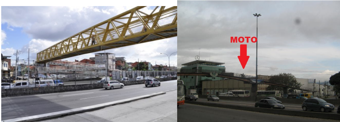
Figure 13. Photos of "Passarelas" Linha Amerela (left) and Avenida Brasil (with a motorcycle going across it - right). From Observatório de Favelas website and Crônicas dumas Viagens Wordpress.
