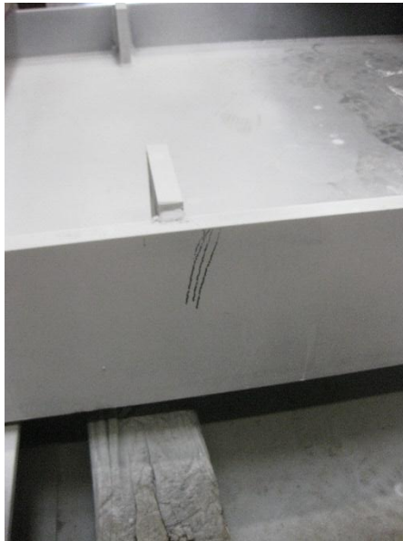
West Flange Outside @ Pick Point
