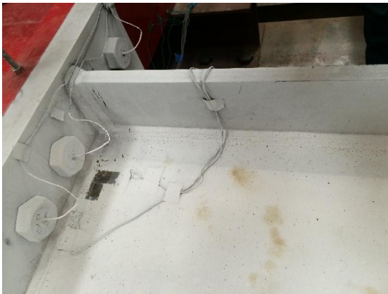
West Flange Inside
