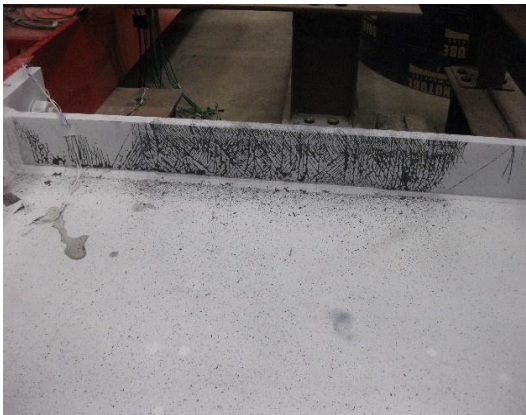
West Flange Inside
