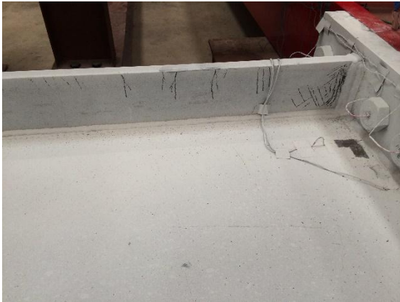
East Flange Inside
