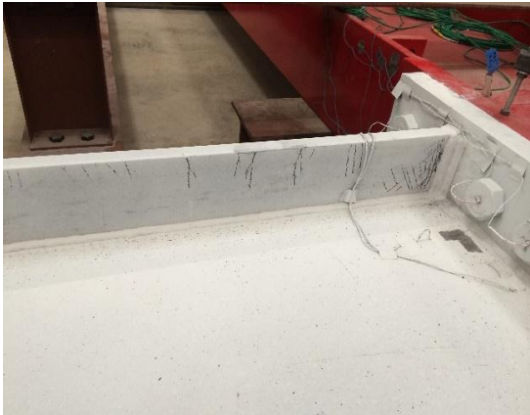
East Flange Inside
