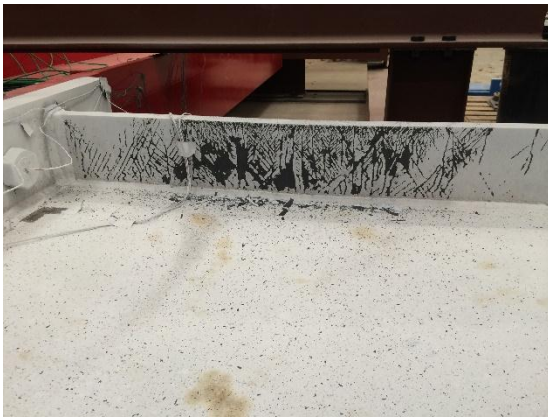
West Flange Inside
