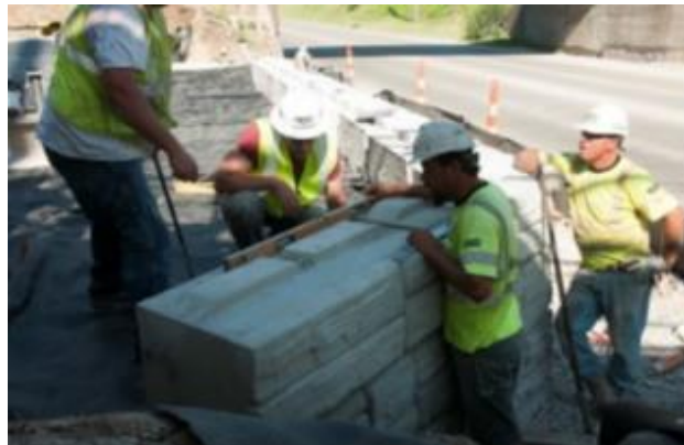
Figure 18: Large wet cast CMU block in Missouri (Bartlett 2015)
