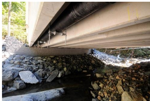
Figure 34: Bottom view of 27 th Street Bridge (Diop et al. 2015)
