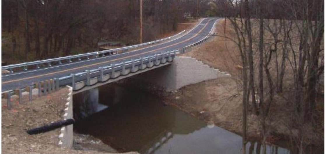
Figure 4: Bowman Road Bridge in Defiance County, OH (Defiance 2016)
