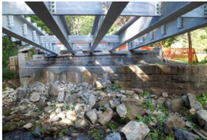
Figure 30: Bottom view of Grove Township / Sportsman Bridge (Alzamora et al. 2015)
