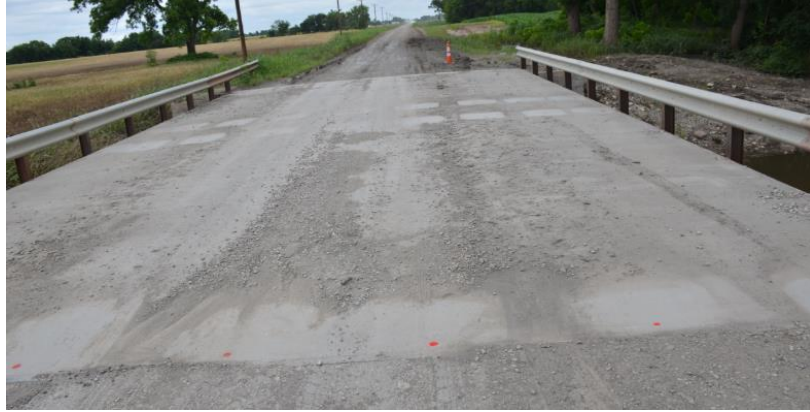
Figure 63: Survey points marked with permanent red paint on Bridge No. 2
