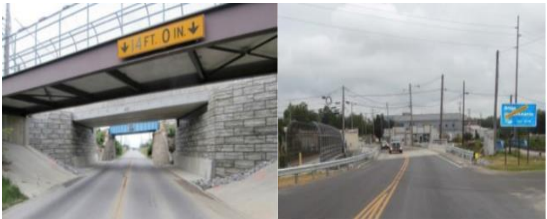
Figure 17: Completed Route B Bridge in Missouri (Bartlett 2015)
