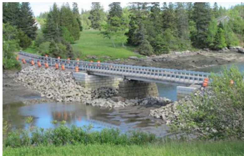
Figure 19: Knox County Beach Bridge in Maine (Alzamora et al. 2015)
