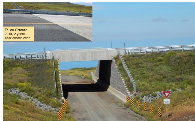
Figure 31: Saddle Road Bridge side view (Alzamora et al. 2015)
