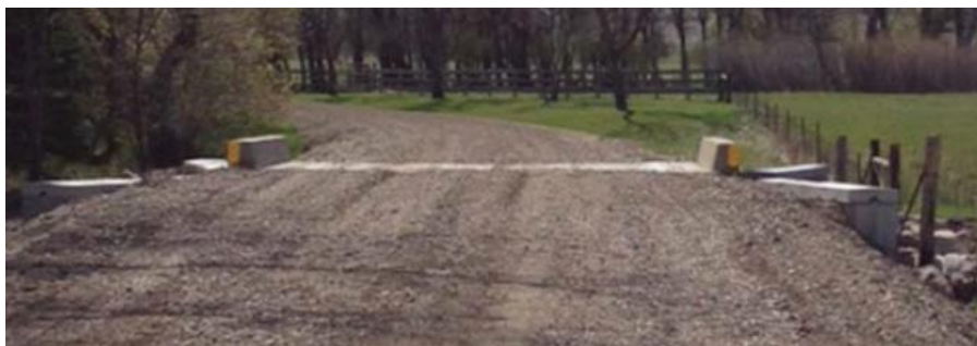
Figure 28: Front view of completed Fergus County Road Bridge (Jenkins 2015)
