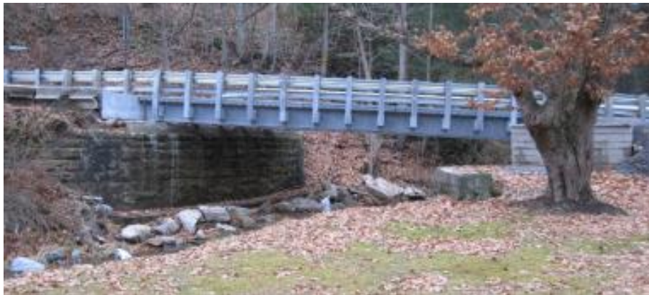
Figure 29: Side view of Grove Township / Sportsman Bridge (Alzamora et al. 2015)
