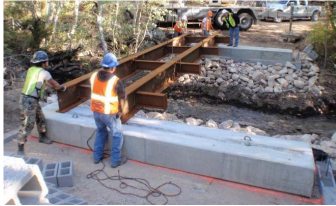
Figure 15: Superstructure Placement (Alzamora 2015)
