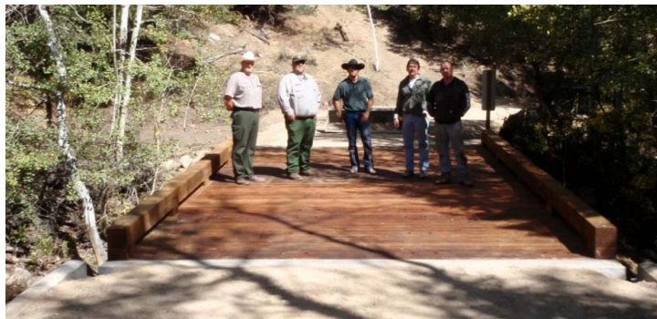
Figure 16: The Strawberry Creek Bridge in Nevada (Alzamora et al. 2011)
