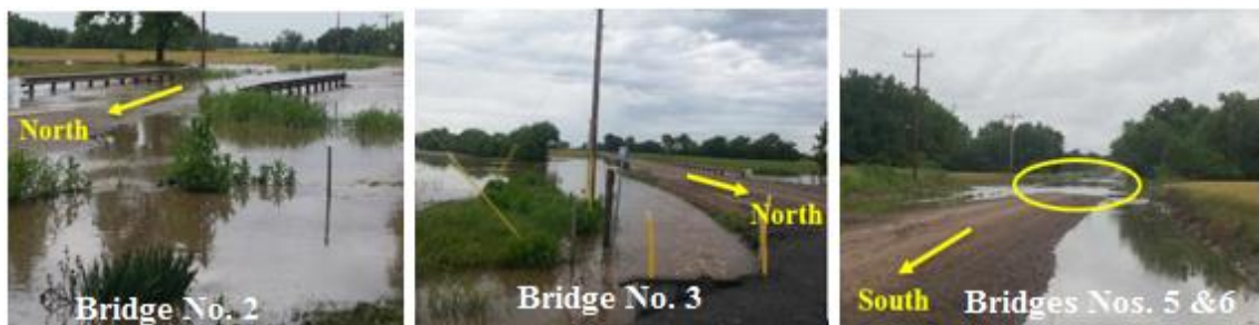
Figure 45: Flooded bridges in Kay County on 05/24/2015; Bridges Nos. 2, 3, 5 and 6 (Photo Courtesy of local residents, Mrs. Curl)
