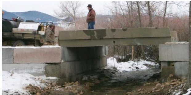
Figure 27: Superstructure placement of Fergus County Road Bridge (Jenkins 2015)
