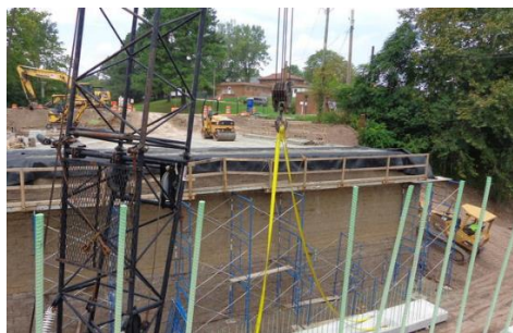
Figure 23: Veterans Administration Hospital Bridge abutment construction (Orders 2013)
