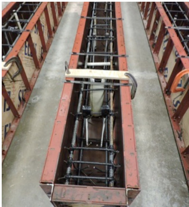
Figure 4.14 FR-SCC Cages in Forms
