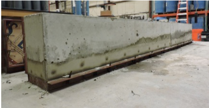
Figure 4.25 FR-SCC Repair Beam Removed from Form
