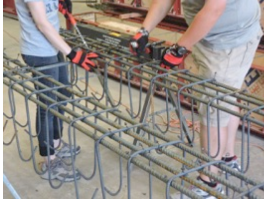
Figure 4.3 Tying Steel Cage Joints
