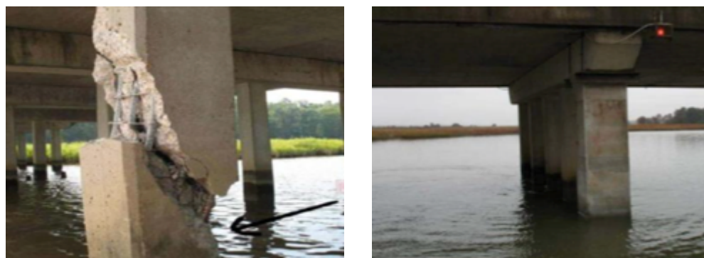
Figure 1.2 SCC Used in the Repair of Bridge Piles
