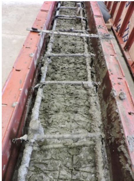
Figure 4.17 Control Concrete Roughened Finish
