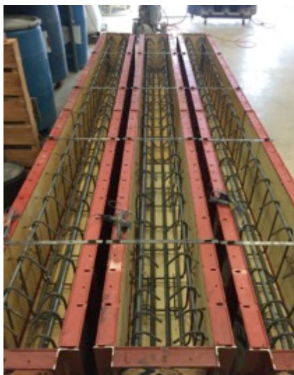
Figure 4.6 Completed Cages Inside Forms
