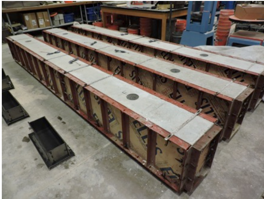
Figure 4.21 FR-SCC Repair Beams Ready for Casting
