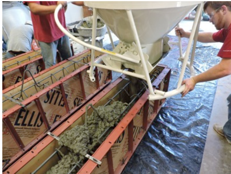
Figure 4.7 Concrete Bucket Filling Forms
