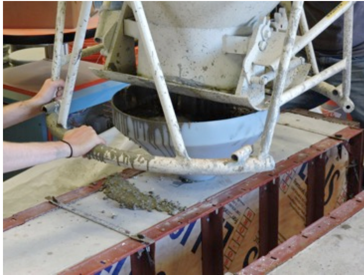
Figure 4.24 Using the Funnel to fill FR-SCC Repair Sections
