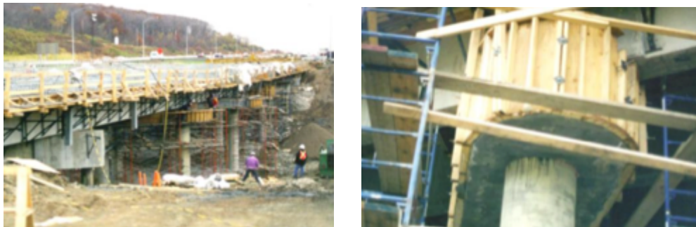
Figure 1.1 SCC Used in the Repair of Bridge Pier Caps
