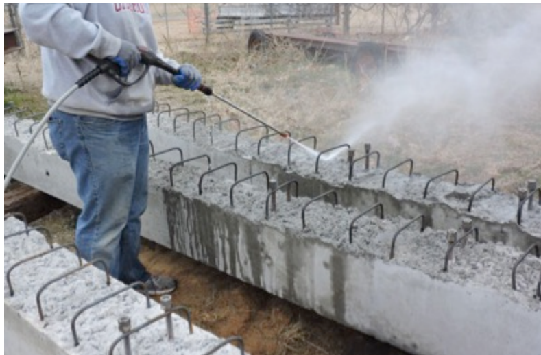
Figure 4.18 Power Washing the Concrete Surface
