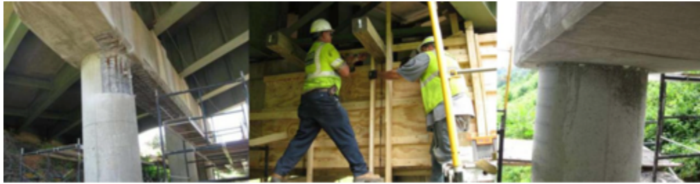
Figure 1.3 SCC Used in the Repair of Bridge Columns and Pier Caps
