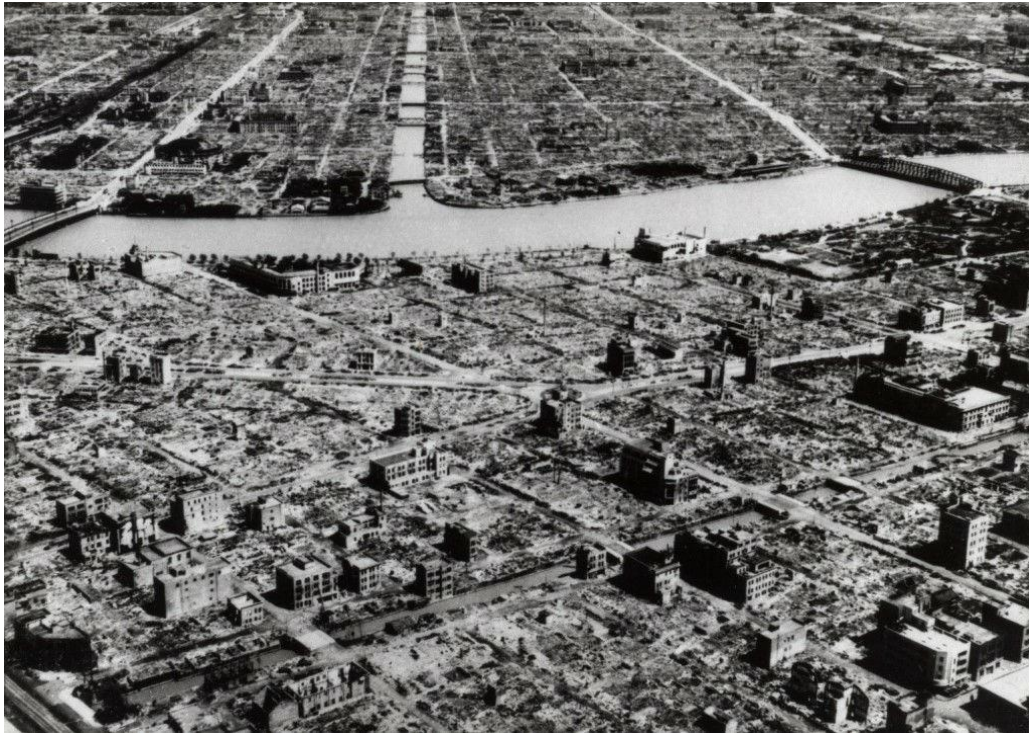
Figure 5: Tokyo's industrial Nihonbashi District after the firebombing on March 10, 1945. Photograph by and courtesy of the U.S. Army.
