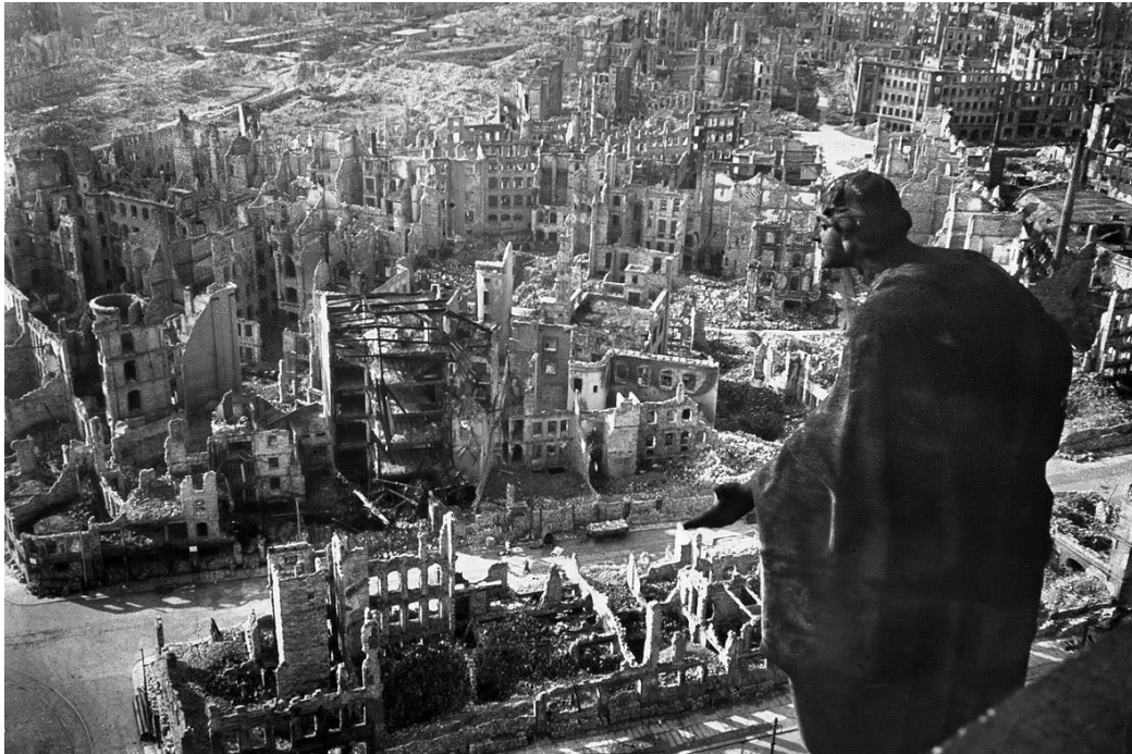
Figure 4: A view from the tower of city hall, Dresden, February 13, 1945. Photograph courtesy of Walter Hahn/AFP/Getty Images.
