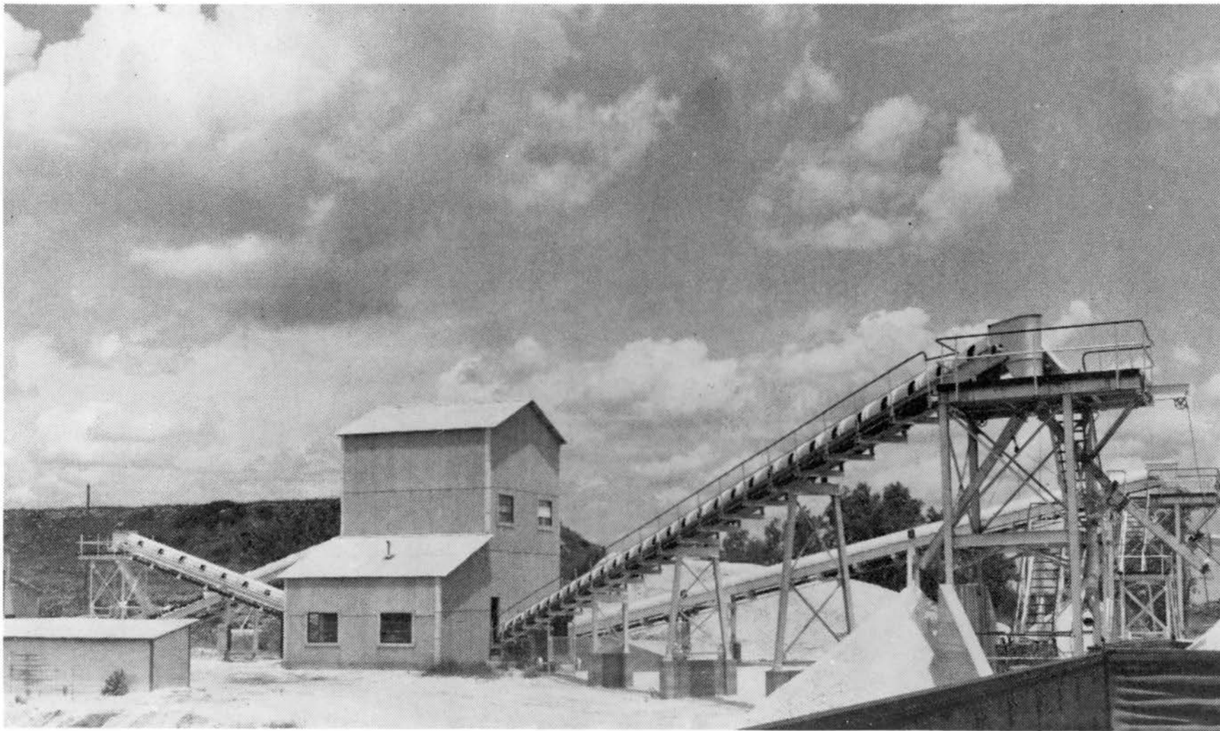
Figure 4. Secondary crushing and screening plant is shown here. Loading platforms drop gypsum into cars. (Courtesy of Universal Atlas Cement Company)
