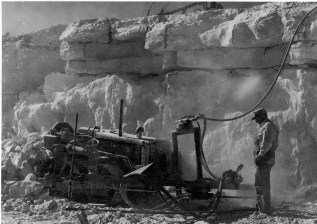
Figure 2. Drilling Operation on Gypsum Ledge (Courtesy of United States Gypsum Company)
